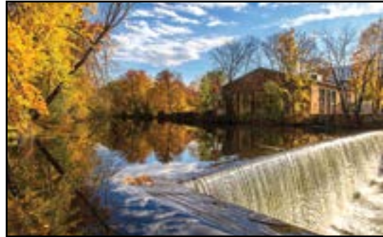
Roundhouse at Beacon Falls
